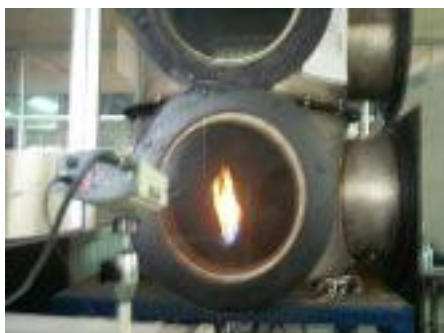
Fig. 2. Burner in operating
